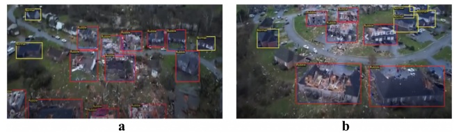
Fig. 11. Model predictions on select frames of the video. These images are from the tornado disasters in Kentucky. In both of these images, the path that the tornado took through this town is clear, because the buildings in the center are labeled as damaged, whereas the ones on the outside are undamaged.
